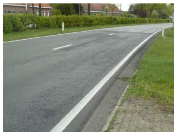
Figure 3.2: Ravelling on Section 5
