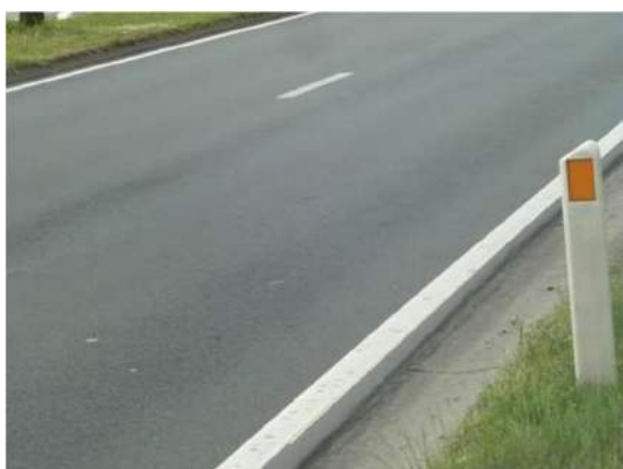
Figure 3.1: Ravelling on Section 2
